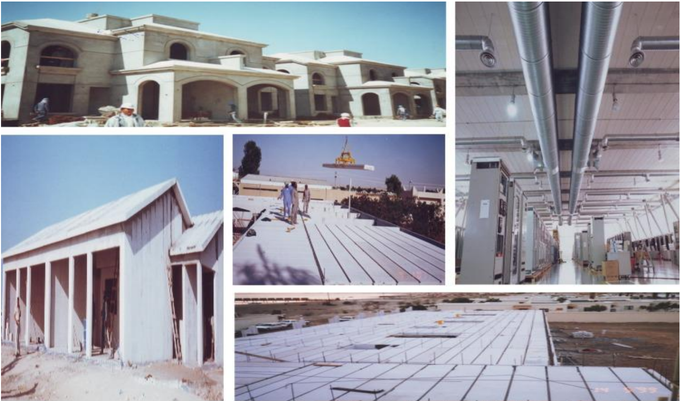
Various applications and construction of Siporex floor/roof slabs
