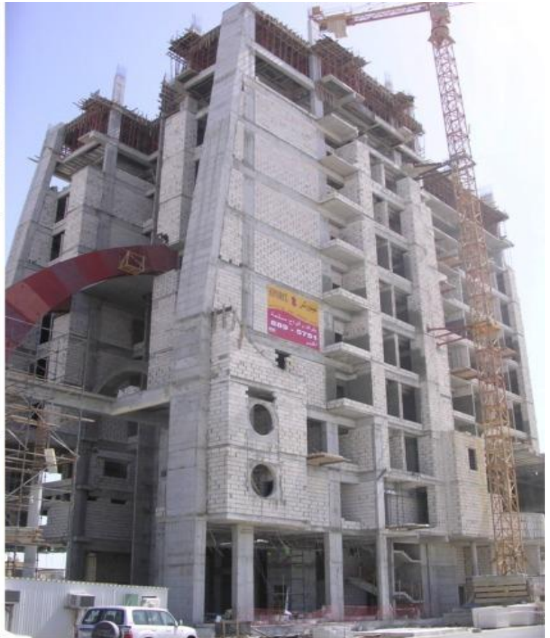
Siporex blocks construction
